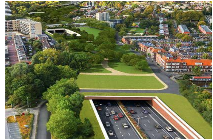
Tunnels for highways in cities
